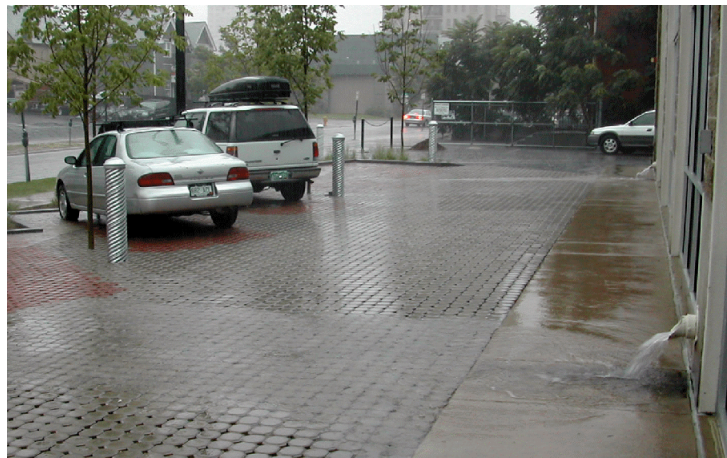
Figure 7. A permeable pavement parking lot in Denver, CO accepts stormwater runoff directly from roof downspouts
