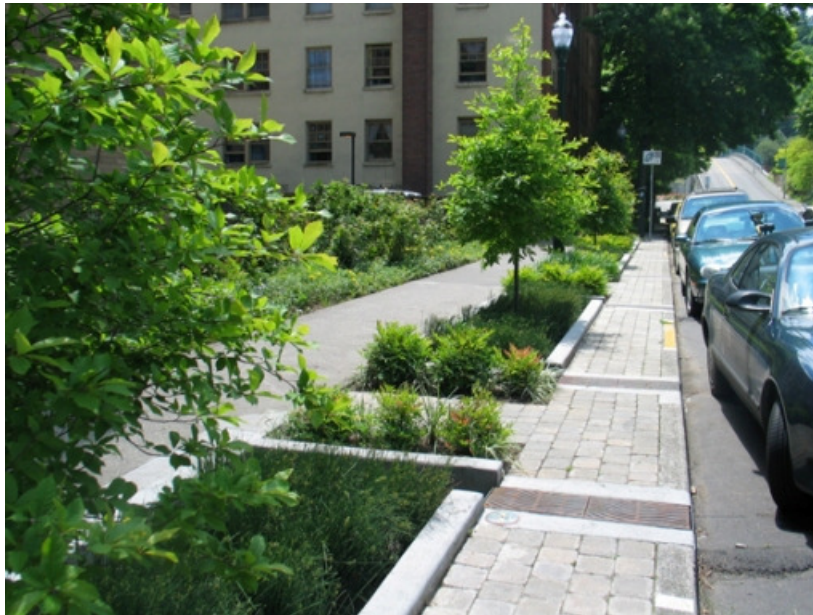
Figure 10. 12th Avenue Green Street featuring bioretention planters, Portland, Oregon
